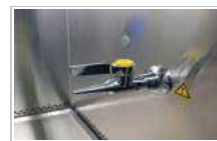
Service Valve (Gas, Air, Vacuum)
